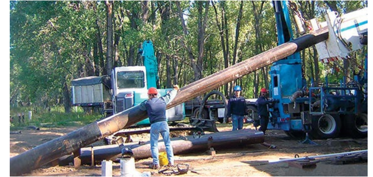
Example: Angle drilled bore injection
