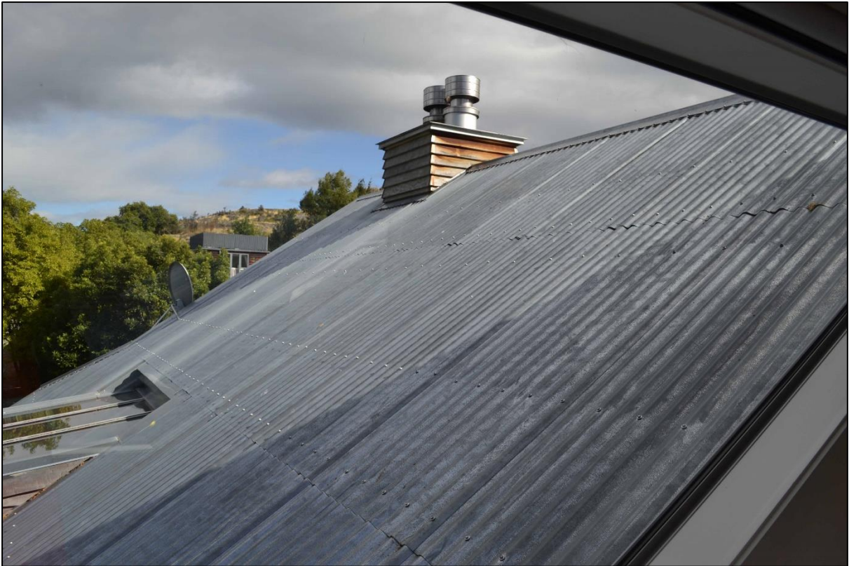
Figure 14. Contemporary turret reflecting original extension to roof line to allow space for wool press.
