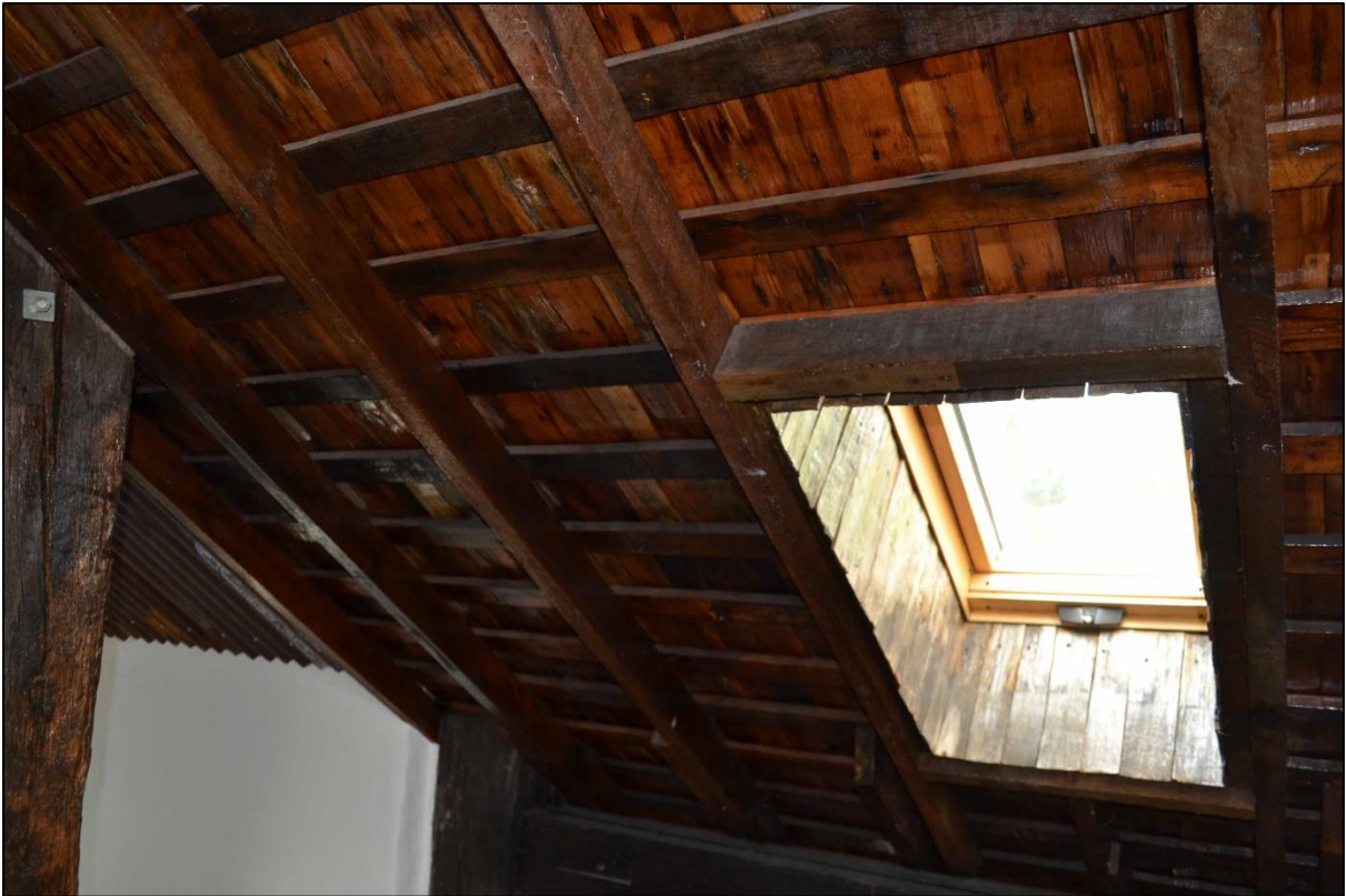
Figure 18. Re-used timber shingles on ceiling interior above main entrance.
