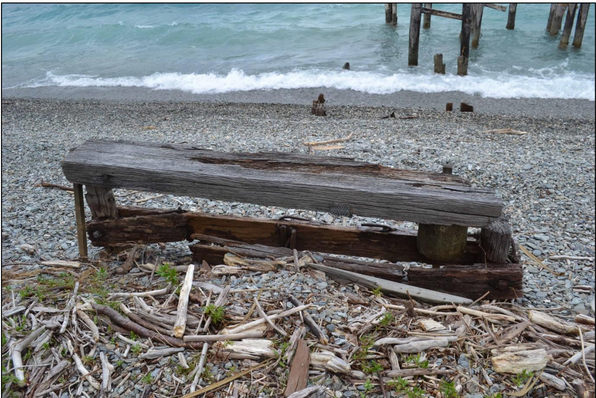
Figure 23. Remains of timber wharf structure.
