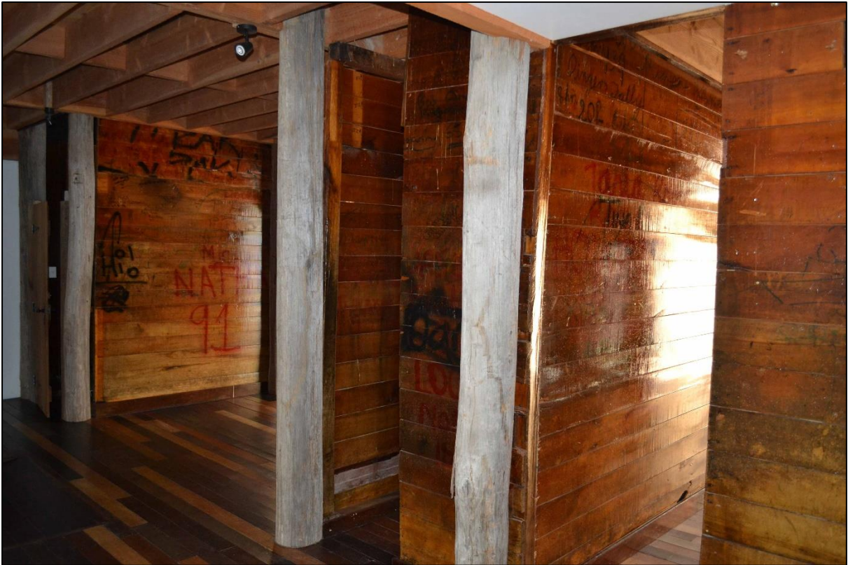
Figure 16. Internal walls of woolshed showing reuse of timber boards as wall linings.
