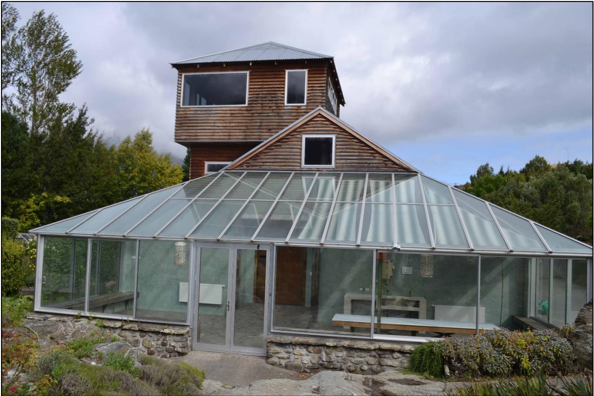
Figure 8. Eastern elevation of woolshed.
