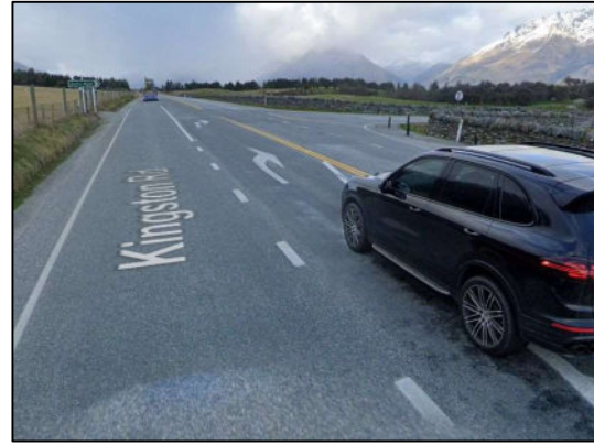
Photo 2.4: SH6 North approach to Maori Jack Road intersection (Source: Streetview)
