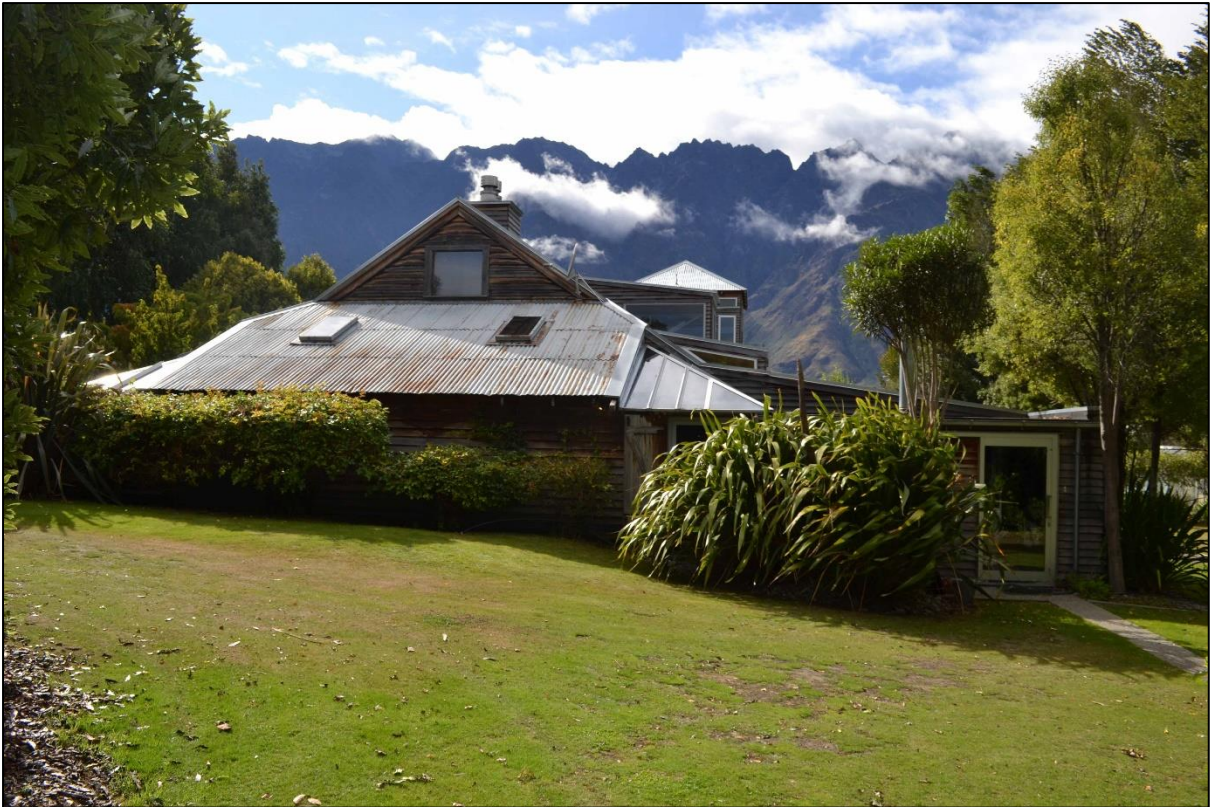
Figure 12. Western elevation of woolshed.
