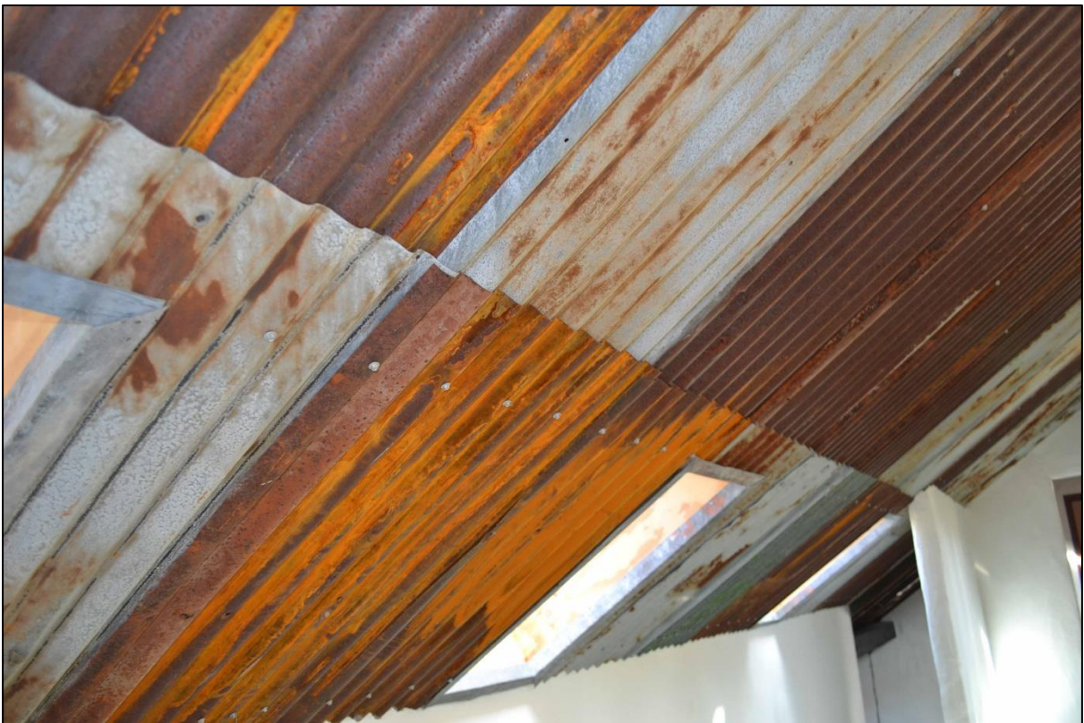
Figure 17. Re-used roofing iron in converted woolshed.
