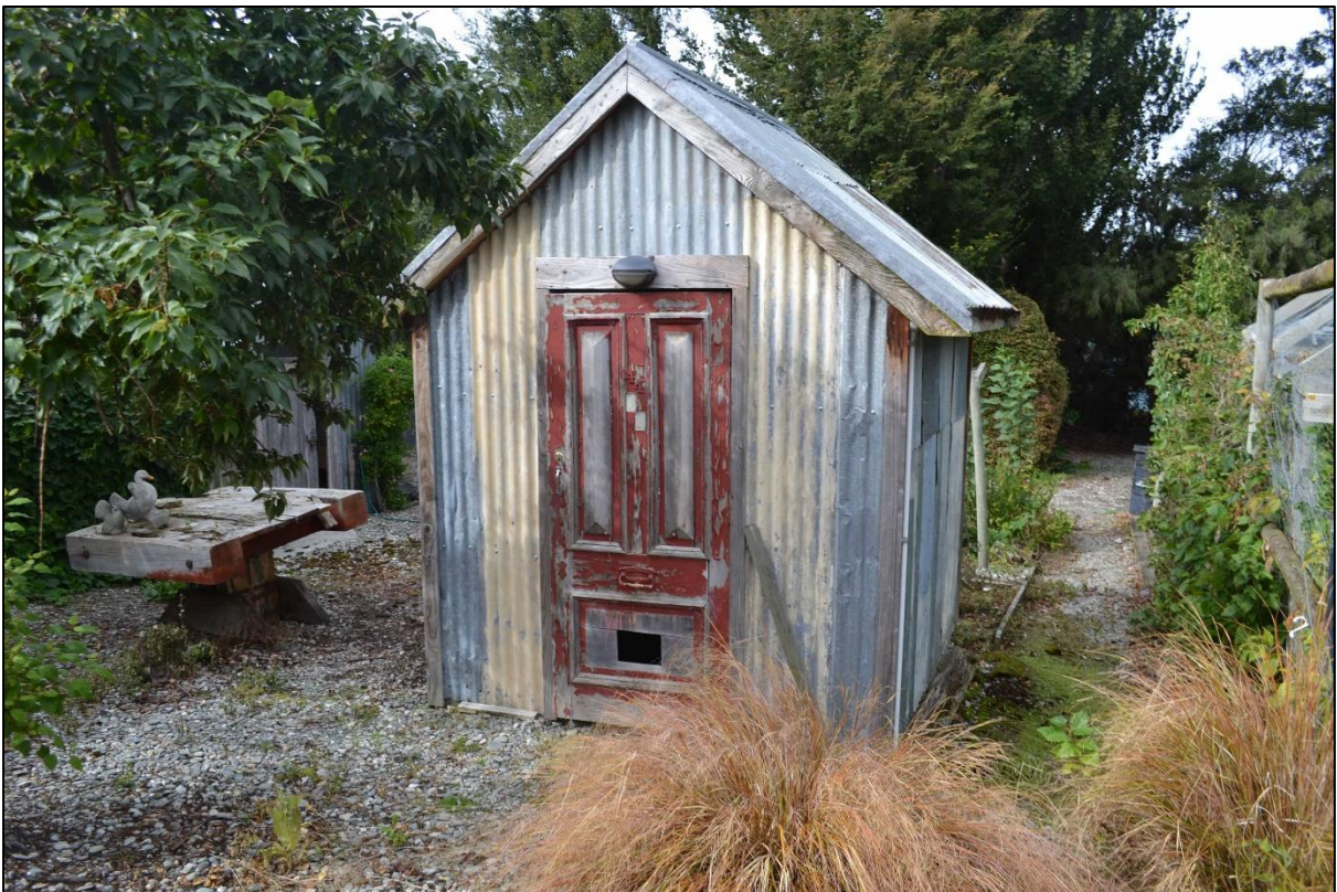
Figure 31. Galvanised iron shed with timber door in garden.
