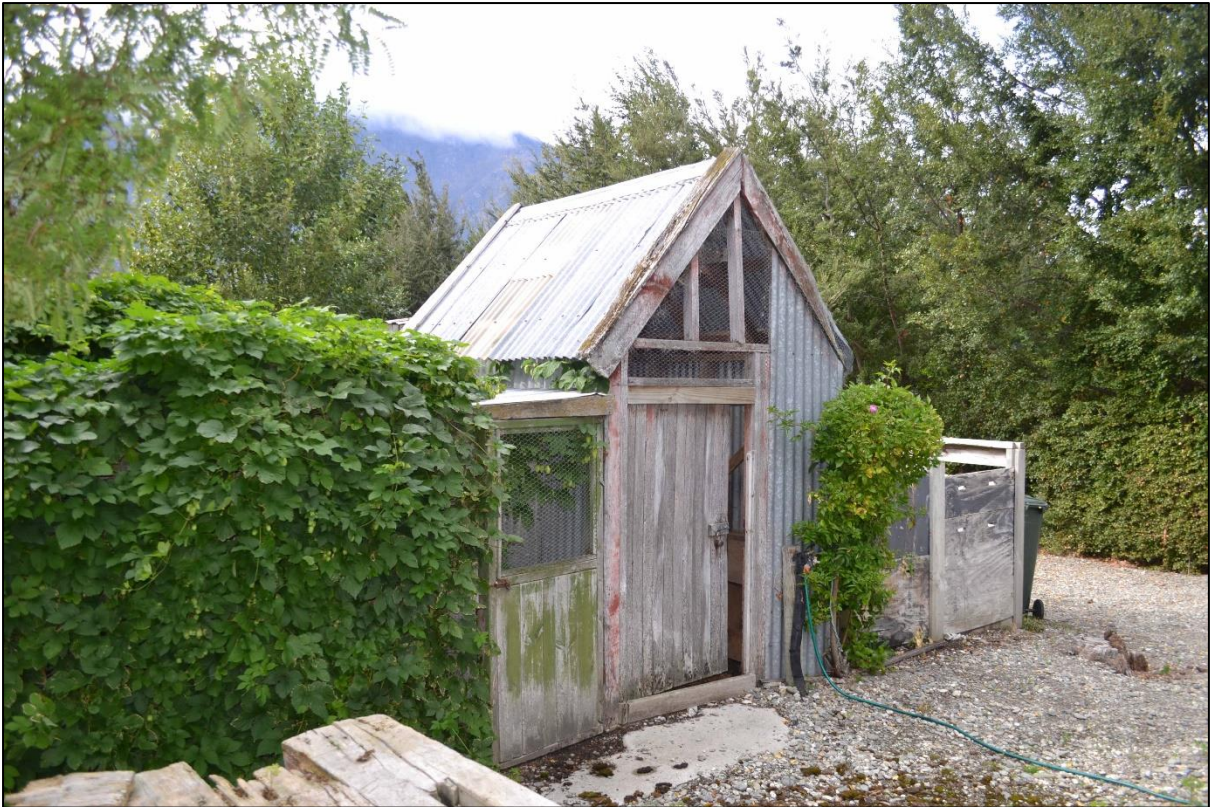
Figure 30. Galvanised iron and timber-framed chicken coop in garden.
