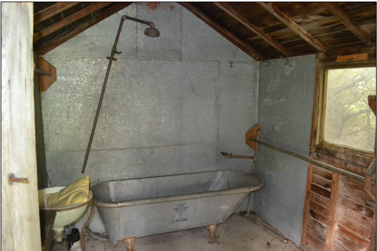
Figure 21. Interior of galvanised iron bathhouse.
