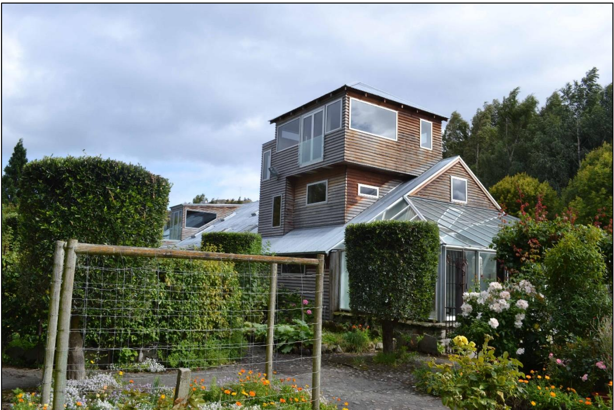
Figure 9. South-eastern corner of the woolshed.
