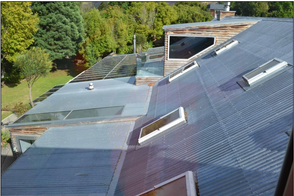
Figure 13. View of woolshed roof showing modern roofing iron and glazing.
