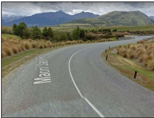
Photo 2.1: Maori Jack Road, close to SH6 intersection (Source: Google Streetview)
