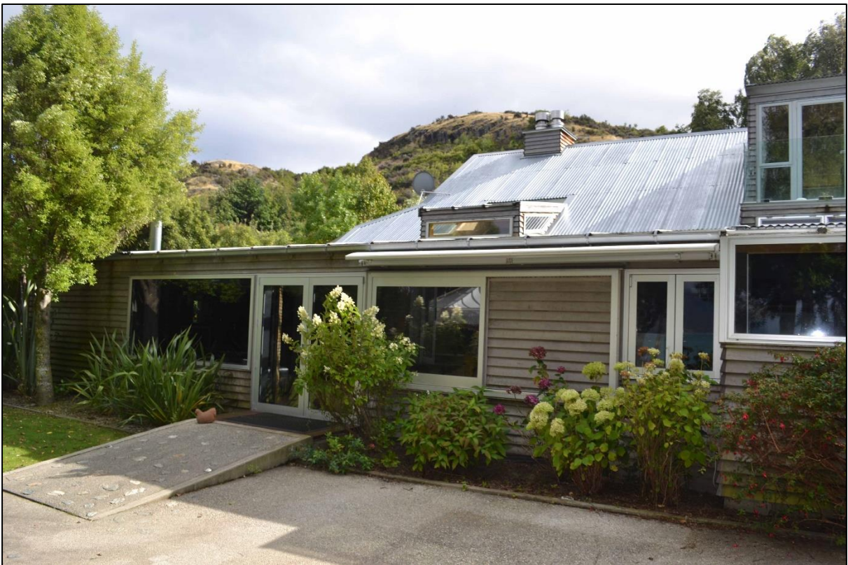
Figure 11. South-eastern corner of woolshed.
