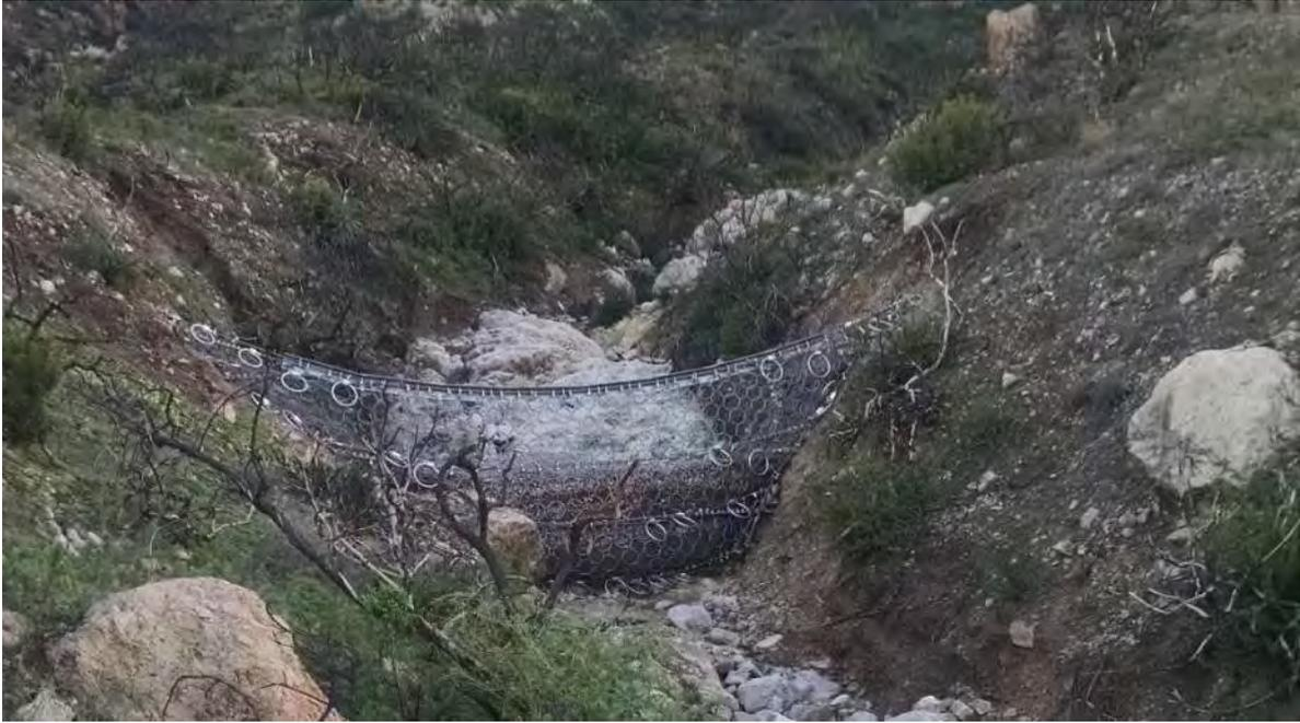
Figure 3 - Example of a debris flow protection fence installed within a stream channel. The fence works to trap large debris and slow flow velocities.
