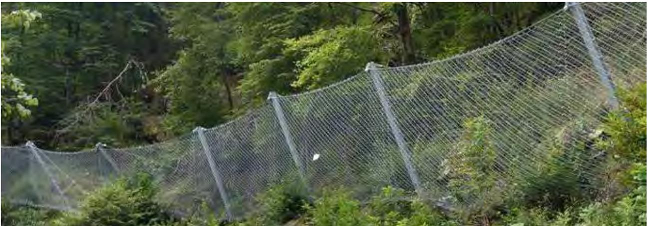
Figure 4 - Example of a rockfall protection fence.
