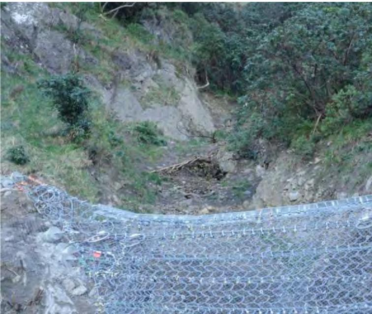
*Looking upslope - VX080-H2 debris flow barrier with 16/3/300 ROCCO ringnet tail. Note abrasion protection on the top ropes.*
