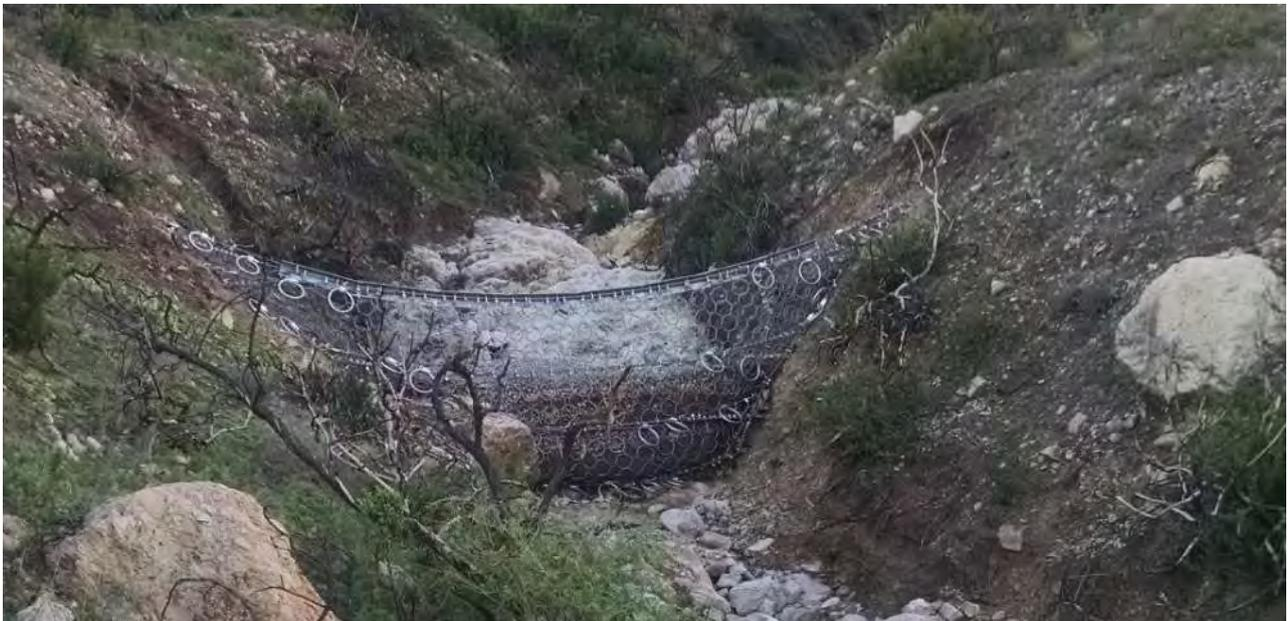
Example of a debris flow fence in a stream channel. The fence works to trap large debris and slow flow velocities.
