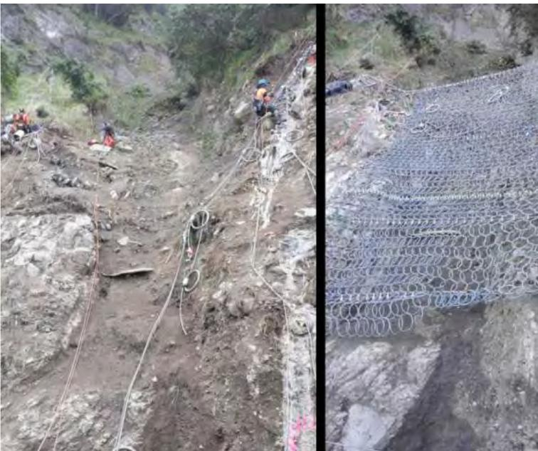
*Looking upslope - VX080-H2 debris flow barrier with 16/3/300 ROCCO® ringnet tail under construction.*
