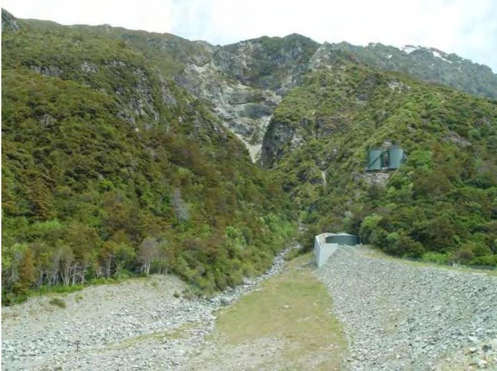
Figure 2 - Example of a debris flow deflection bund installed at Aoraki/Mount Cook Village (source GNS Science, 2017)
