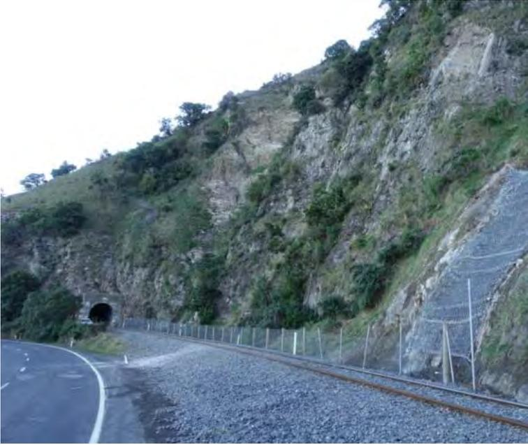
*Looking South - VX080-H2 debris flow barrier with 16/3/300 ROCCO® ringnet tail.*
