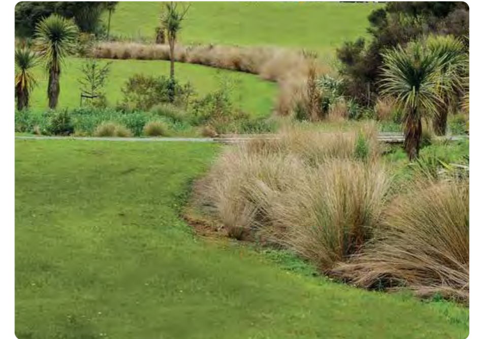
Stormwater swales with native planting and pathways winding across and around.
