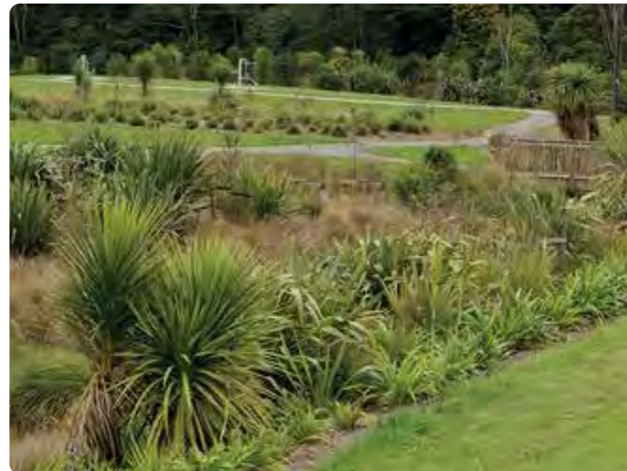
Stormwater retention areas with native planting integrated with pathways.
