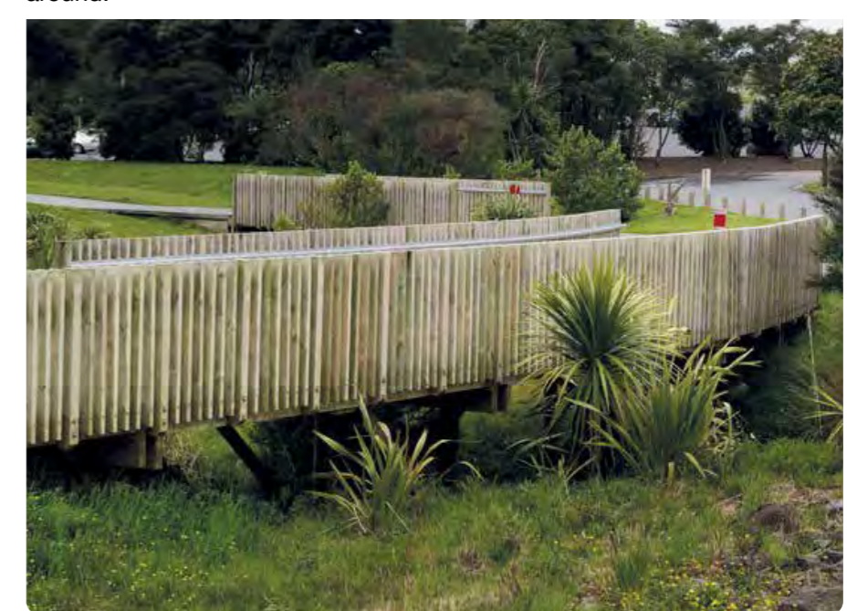
Stormwater retention pond with native planting and walking paths.
